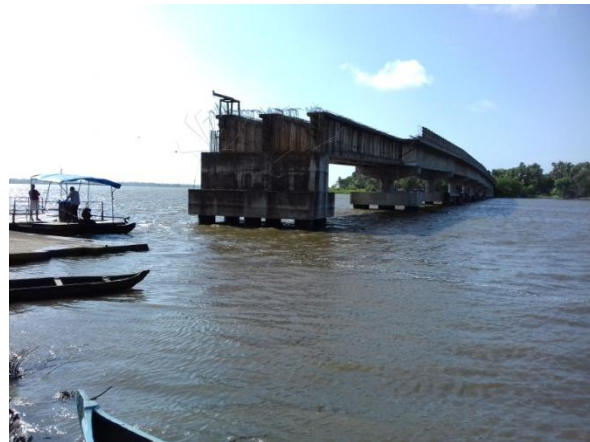
Bridge from the Valiya Kadamakudy end
