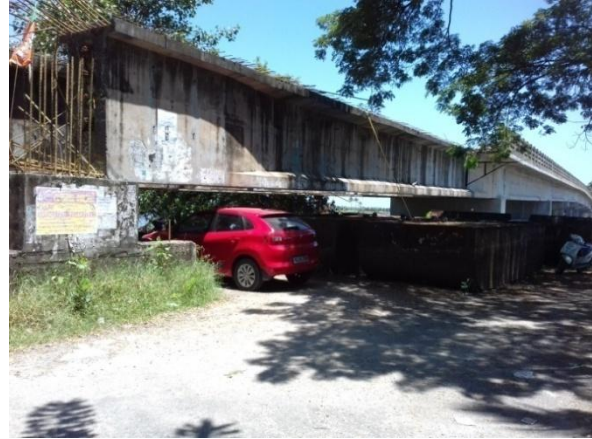
Bridge landing in the Chathanad side
